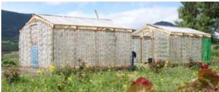
Two 'greenhouses' built with recycled plastic bottles where the Association de la Rosa de Coyhaique will grow roses
